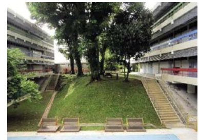
Previously, there was a sloping area and stairs in place of the ramp.
